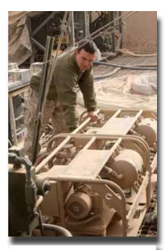
Lance Cpl. Andrew C. Grencer, a water purification technician with Utilities Platoon, Service Company, 8th Engineer Support Battalion, 1st Marine Logistics Group (Forward), turns on a water pump at Forward Operating Base Nolay in Helmand province, Afghanistan, Dec. 5, 2010. Water purification technicians with 8th ESB provide laundry and shower services for Marines with 3rd Battalion, 5th Marine Regiment, 1st Marine Division (Forward), who operate from the FOB. Photo: Lance Cpl. Kenneth C. Jasik
